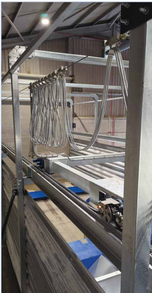
Top Loader fuel store - 90m3 capacity
