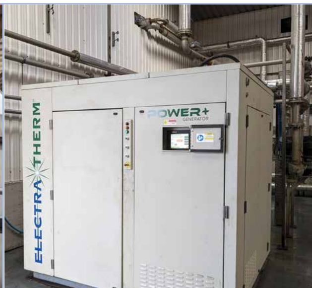
Electratherm 4400 O.R.C (Electrical generation)
